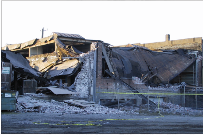
Photograph showing partial collapse of an unreinforced masonry building in the SODO neighborhood of Seattle, Washington, caused by the 2001 magnitude 6.8 Nisqually earthquake. Photograph by Kathy Troost, University of Washington, used with permission.
