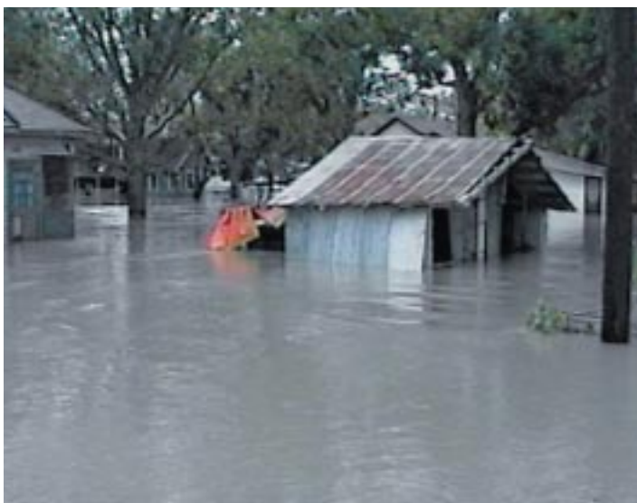
View of structures inundated by the Guadalupe River at Victoria, Tex. (From video by M.W. Sunvison, D.S. Brown, and B.L. Petri, U.S. Geological Survey.)
