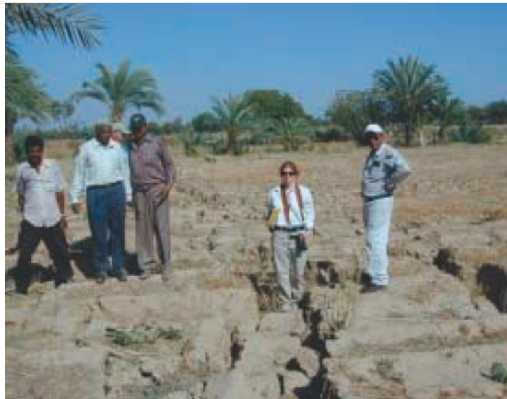
Figure 4. Ground failure from the Bhuj earthquake most likely resulted from shaking, as the soil mass cracked and slid down the almost imperceptibly sloping ground surface. No permanent changes to the topography directly related to faulting have been identified. The flat terrain suggests that few shallow earthquakes have occurred here previously and (or) that the processes leading to frequent (geologically) large earthquakes have not been going on for very long.
