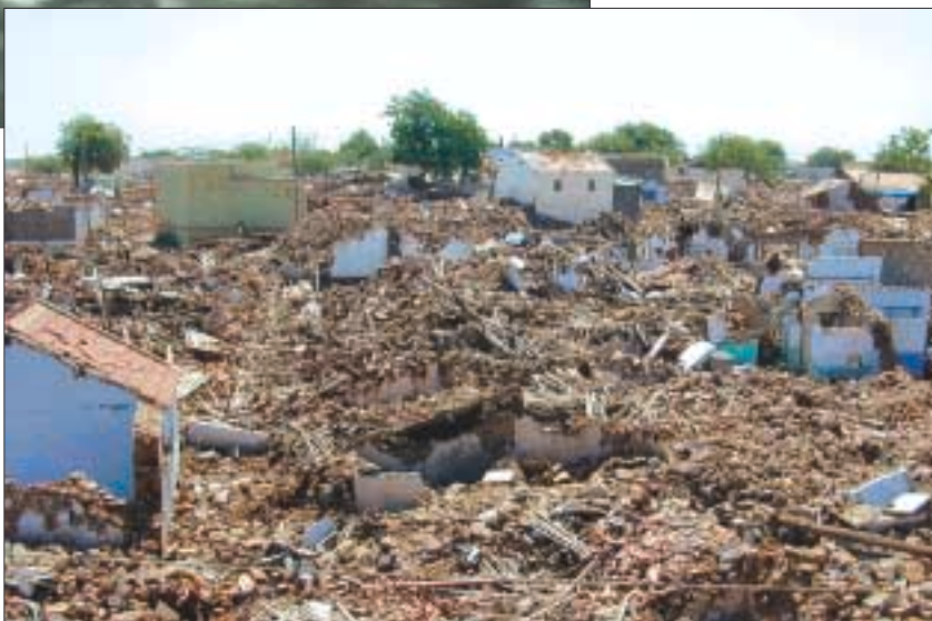
Figure 6. Collapsed houses in the town of Ratnal, in the epicentral region of the Bhuj earthquake. The almost total devastation may, in large part, be attributed to construction methods that have no resistance to earthquake shaking.
