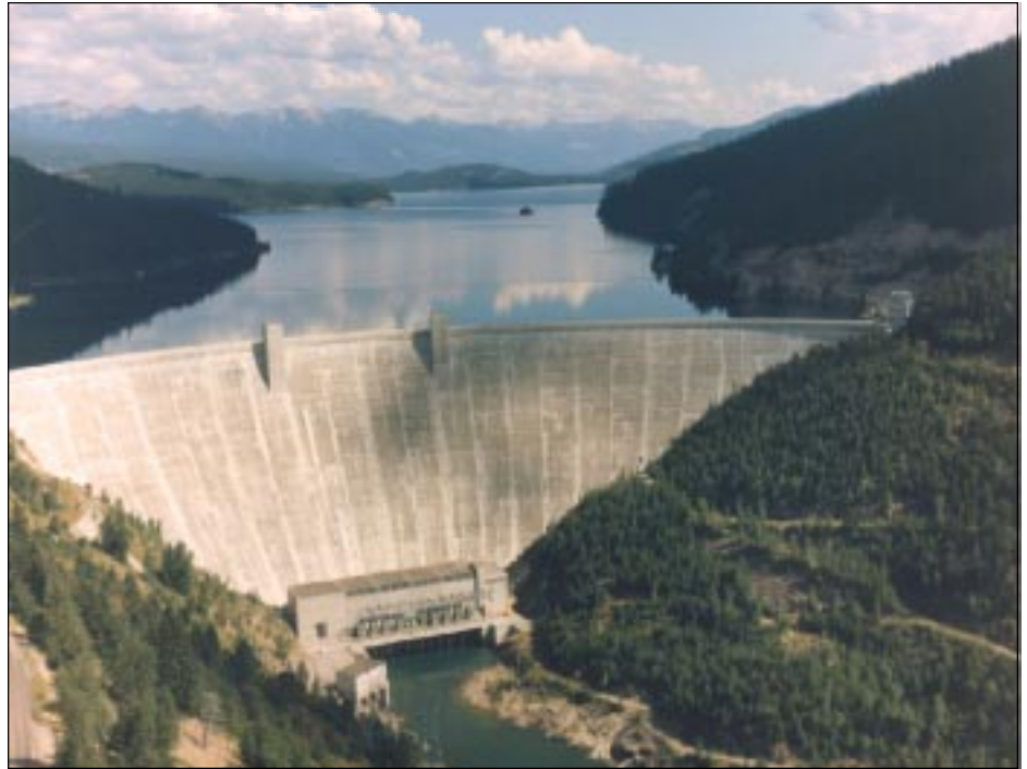
Figure 5. Hungry Horse Dam, Montana, is a thick-arch structure that was built between 1948 and 1953 with concrete containing 120,000 metric tons of fly ash. The use of coal fly ash in cement and concrete displaces portland cement. Photograph from the U.S. Bureau of Reclamation.
