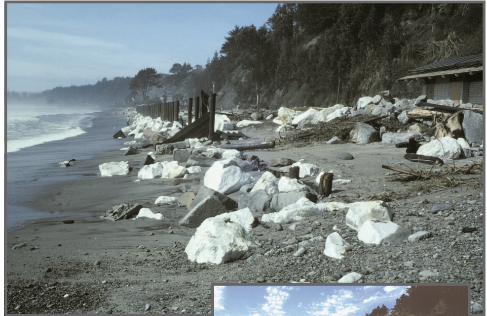
Waves generated by severe winter storms during the 1982-83 El Niño destroyed the wooden seawall at Seacliff State Beach on California's Monterey Bay. The barrier of large stones that had been emplaced seaward of the wall was also scattered by the waves (photo above). The photo at right, taken 2 years after these storms, shows the replacement seawall and rebuilt beach. This seawall remained intact during the 1997-98 El Niño.
