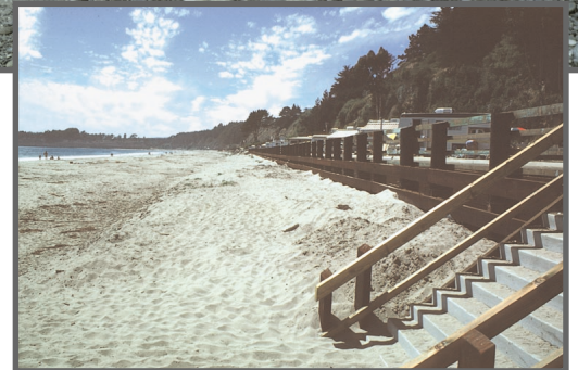
Waves generated by severe winter storms during the 1982-83 El Niño destroyed the wooden seawall at Seacliff State Beach on California's Monterey Bay. The barrier of large stones that had been emplaced seaward of the wall was also scattered by the waves (photo above). The photo at right, taken 2 years after these storms, shows the replacement seawall and rebuilt beach. This seawall remained intact during the 1997-98 El Niño.
