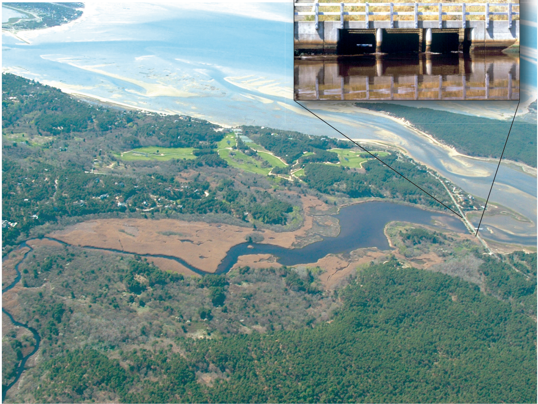
Figure 12. Tide-control structures open at low tide to allow freshwater to flow to the coast and close at high tide to prevent saltwater from flooding original salt marshes, such as in the Herring River Basin. The ecologically damaging effects of tide restrictions are prompting tide-restoration projects on Cape Cod and throughout the world.
