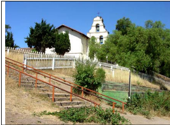
Figure 2-8. The San Juan Bautista Mission. The trace of the San Andreas Fault runs along the foot of a historic grandstand (painted green) along the "El Camino Real" (at the base of the stairs). The historic road runs along the San Andreas Fault scarp through the northeast side of town.
