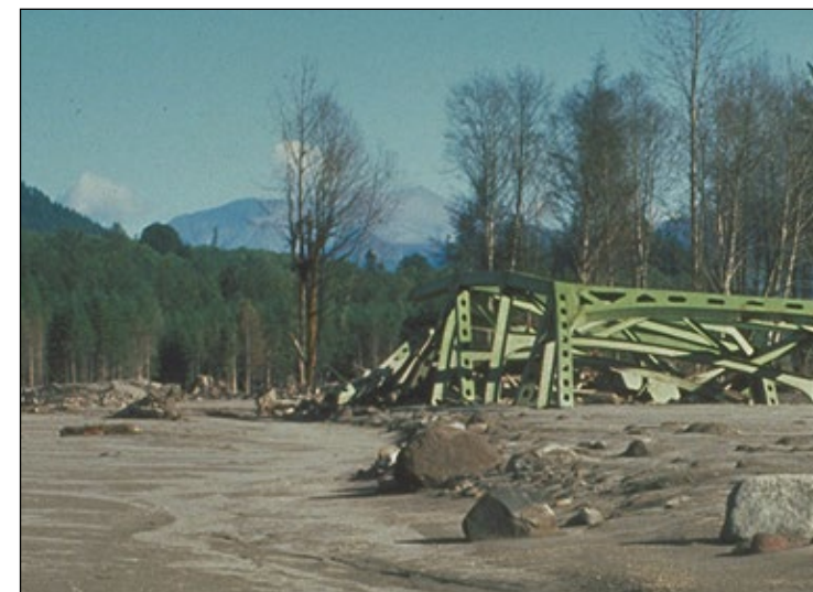
Bridge destroyed by lahar in North Fork Toutle River during eruption of Mount St. Helens, May 18, 1980. Photograph by Richard Waitt, U.S. Geological Survey.
