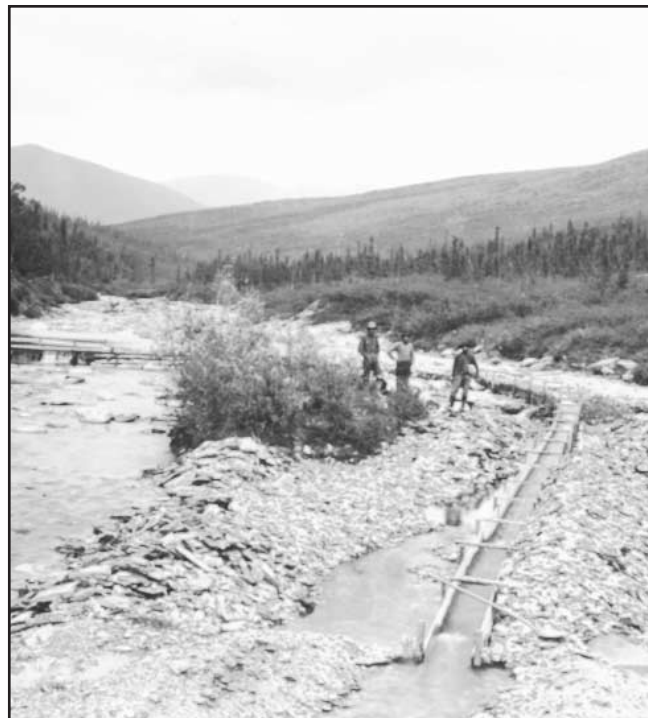
Recovering gold in a long sluicebox. Gold-bearing gravels are shoveled into the upper end of the sluiceway; a series of riffles set across the bottom of the box traps the gold. Myrtle Creek, Alaska, circa 1900.
