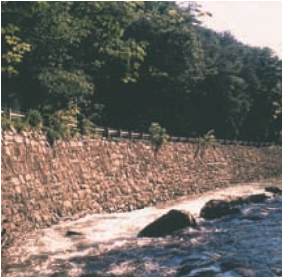
Block-field sandstone retaining wall on Passage Creek.
