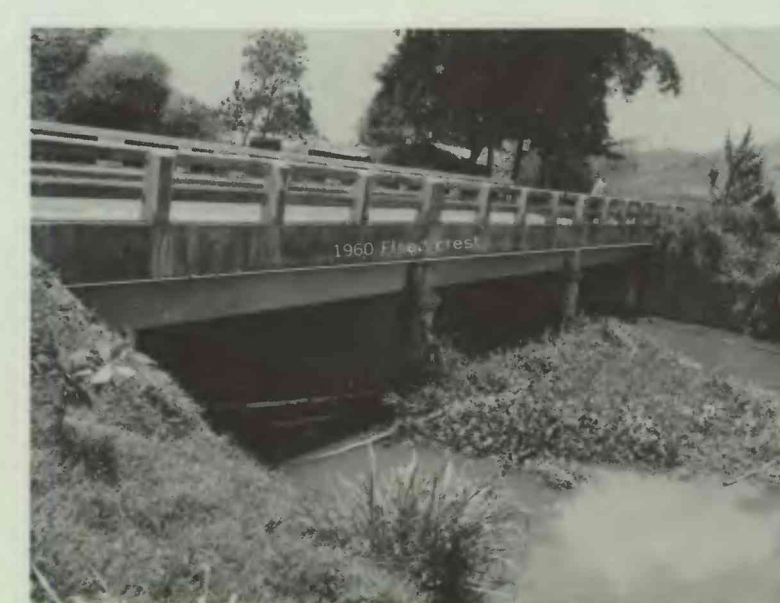
FIGURE 2.—Highway PR-3 bridge spanning Río Guayanés. The 1960 flood (shown by white line) reached a crest 0.5 meter below the roadway level.
