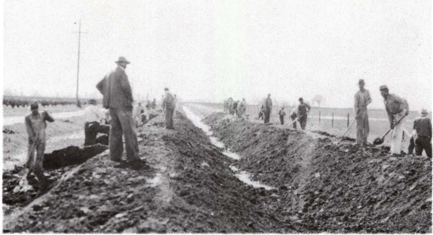
Preparing a canal for concrete lining. (Woodbridge Irrigation District.)
