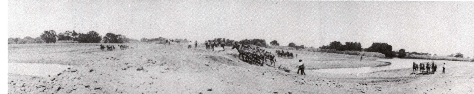
Fresno scrapers and mule teams digging canal. The workers were paid in gold. (Patterson Township Historical Society.)
