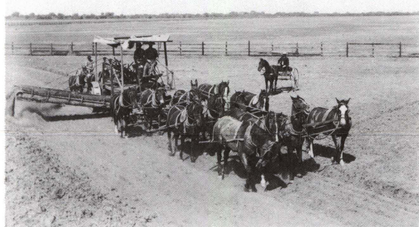
Ditching machine used in the late 1800's and early 1900's to build ditches and levees or other embankments. One person on one side was centered to the other side by a rope. Twelve horses and mules are pulling and four are passing. Moving 1,000 cubic yards per day was a good average, costing about 2 cents per cubic yard. (City of Bakersfield, Department of Water.)
