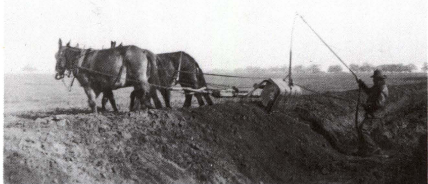
A mule-drawn Fresno scraper dumping a load of dirt scarified from a canal bottom. (Woodbridge Irrigation District.)
