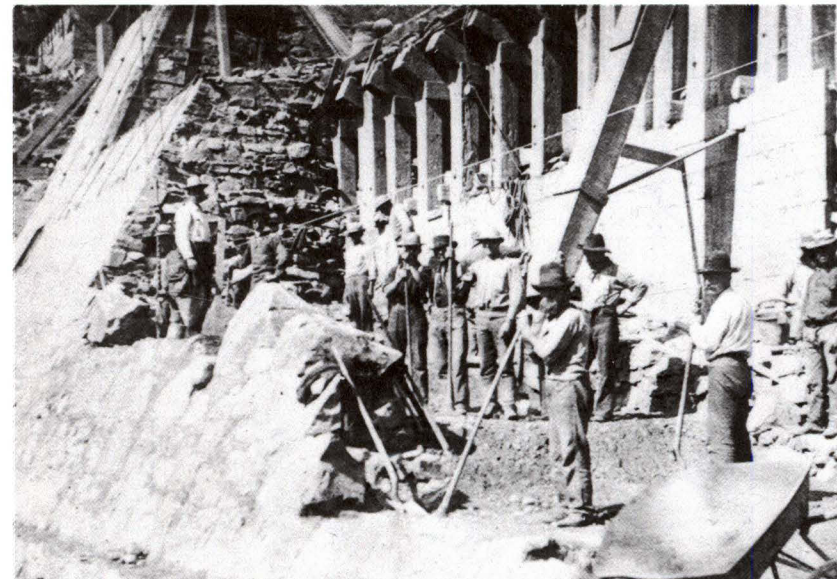
North Fork Dam (no longer in existence), manually built of native rock and concrete in the early 1900's, on a canal adjacent to the main stream. The location was the same as the proposed Auburn damsite. (San Juan Suburban Water District.)
