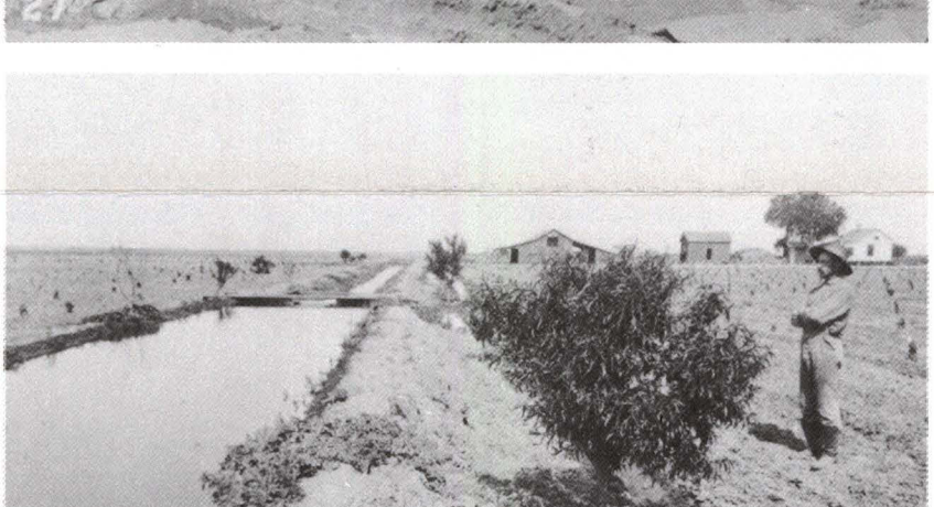
Manually dug ditches in Rosedale Colony, Kern County, in 1890. (City of Bakersfield, Department of Water.)
