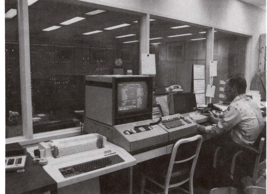
Electronic control board and computers in Sacramento used by the Central Valley Project of the U.S. Bureau of Reclamation to distribute water for irrigation. Flow control and safety control. The release of water from reservoirs according to user demand is simple in theory, but in practice it requires technical personnel monitor river and reservoir data that feed out on the same board seen in the background. The control center is linked to the field. (U.S. Bureau of Reclamation, the California Department of Water Resources, the U.S. Army Corps of Engineers, and the Federal-State River Forecast Center. (U.S. Bureau of Reclamation.)
