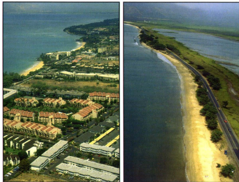
Small pocket beaches of Kihei (left) give way to a long, narrow beach fronting Kealia Pond (right) where rapid sea-level rise and chronic erosion are threatening the coastal road.
