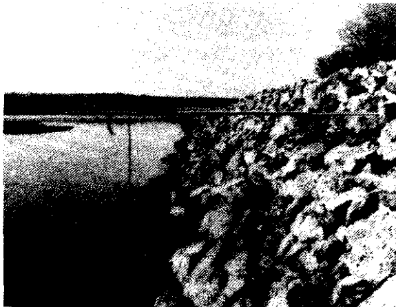
FIGURE 5 VIEW ALONG SLOPE PROTECTION BELOW THE THICK HORIZONTAL BLANKET. SURVEY ROD SHOWS LOCATION OF THE BASE OF THE TOE
