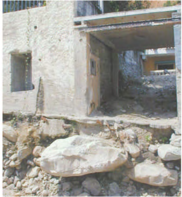
Figure 7. House and garage on Caraballeda fan with exposed foundation showing old debris flow deposit.
