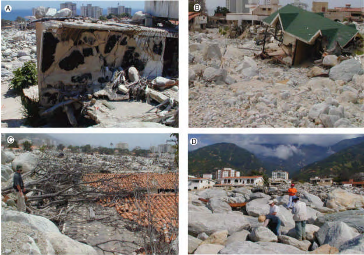
Figure 5. Debris flow deposits on the Caraballeda fan (A) House with 1-m diameter boulders on roof. (B) Concrete house rotated off foundation by debris flow (C) View across debris fan; tiled surface on right is top of one story home. (D) View up debris fan looking towards San Julián Canyon.
