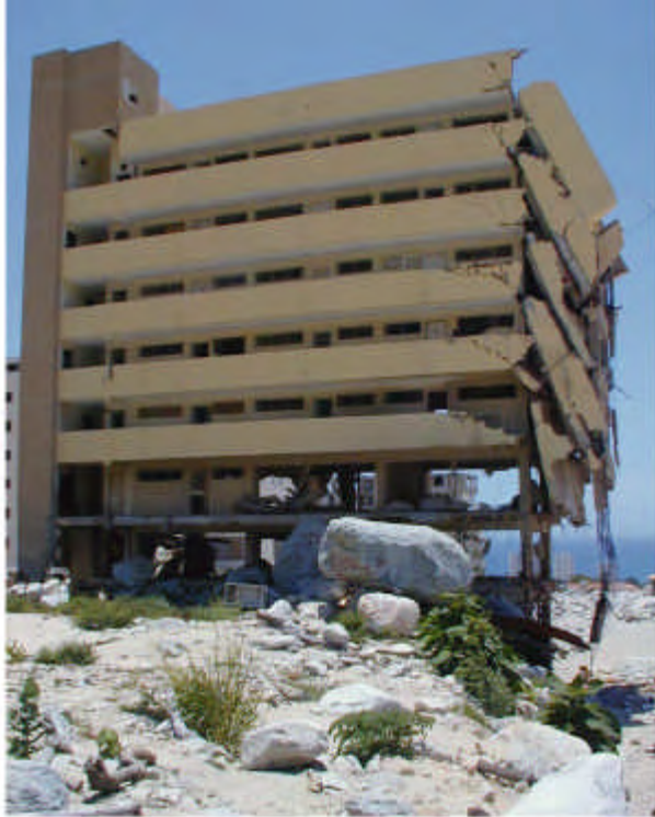
Figure 6. Apartment building damaged by debris flows Caraballeda. Note collapsed apartments and boulders on floor of second story.
