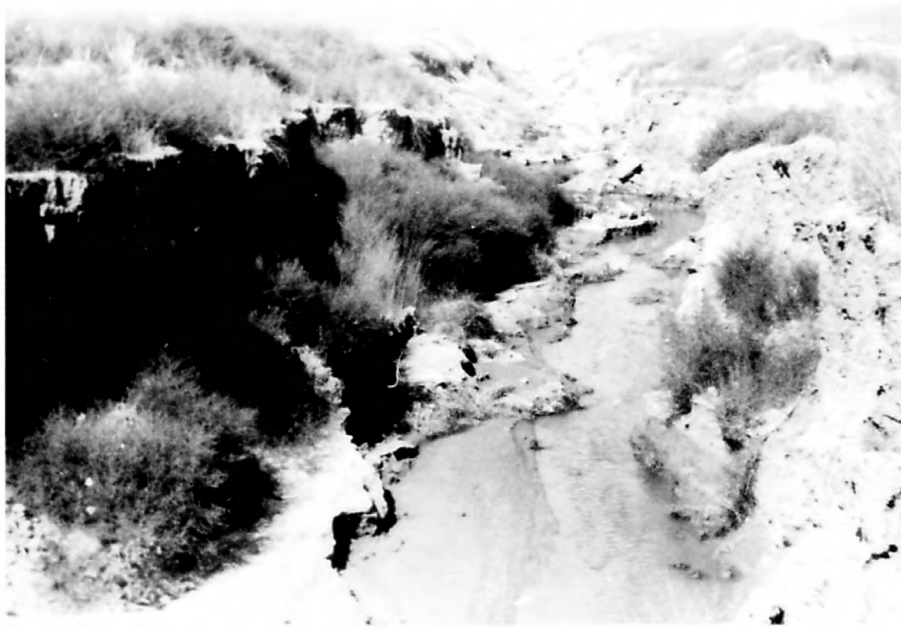
View of drain into Five Mile Creek on the Riverton Project This drain eroded to its present depth from its original depth of not over four feet in less than three years.
