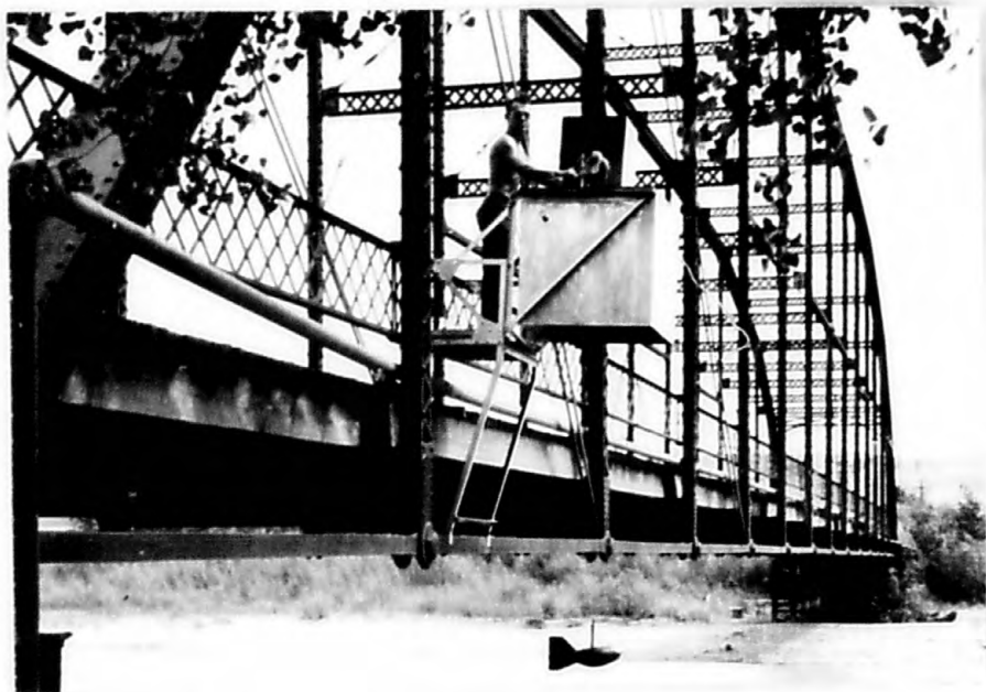
US D-43 sediment sampling installation Bighorn River at Thermopolis, Wyoming
