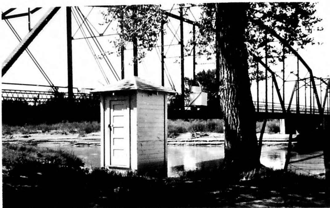
US D-43 sediment sampling installation and water-stage recorder shelter. Bighorn River at Kane, Wyoming.
