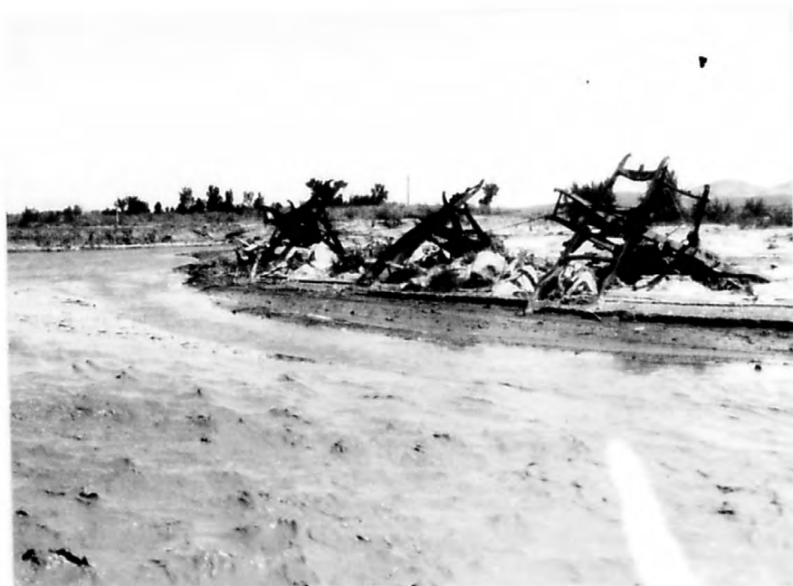
View upstream near the mouth of Cottonwood Creek. Steel revetments now on inside of meander were placed on the outside of the meander in 1937.
