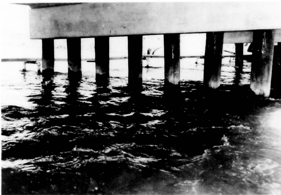
B. View of section C looking upstream from right abutment at section D. Baffles of turbulence-inducing structure causing riffles in foreground.
