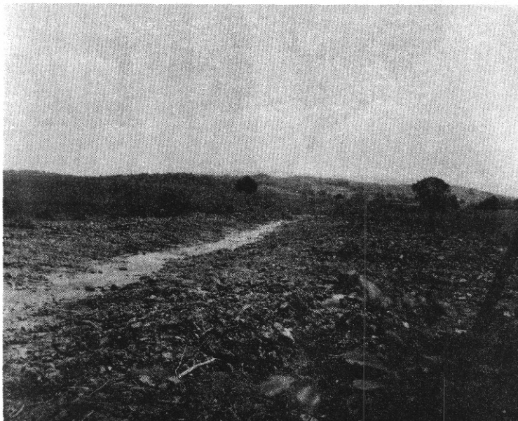
Figure 18. - Channel straightening job immediately after completion in May 1956.
