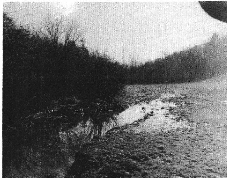
Figure 7. - East Branch Bixler Run showing buildup of a natural dam to possibly change the course of the stream.
