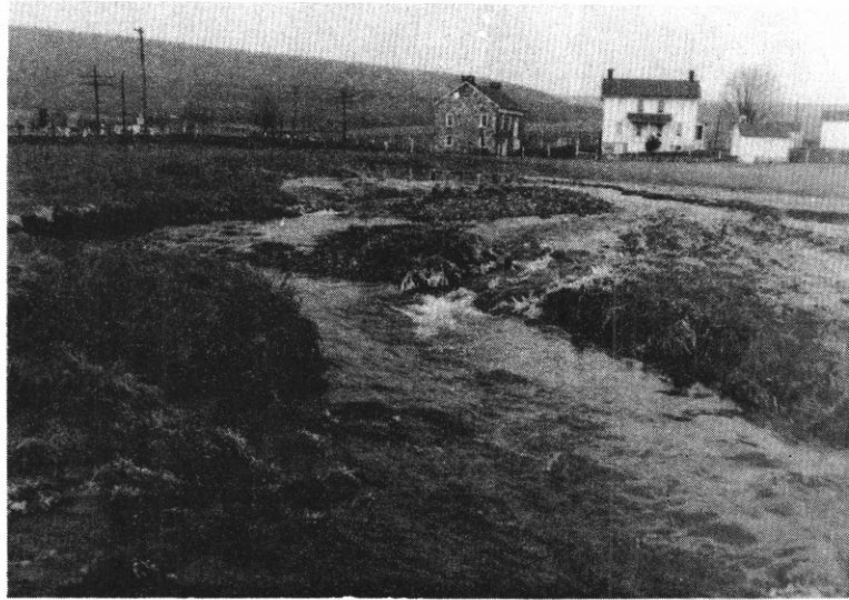
Figure 6. - Bixler Run at Kistler showing rock and gravel fill causing widening and eventual splitting of the channel.
