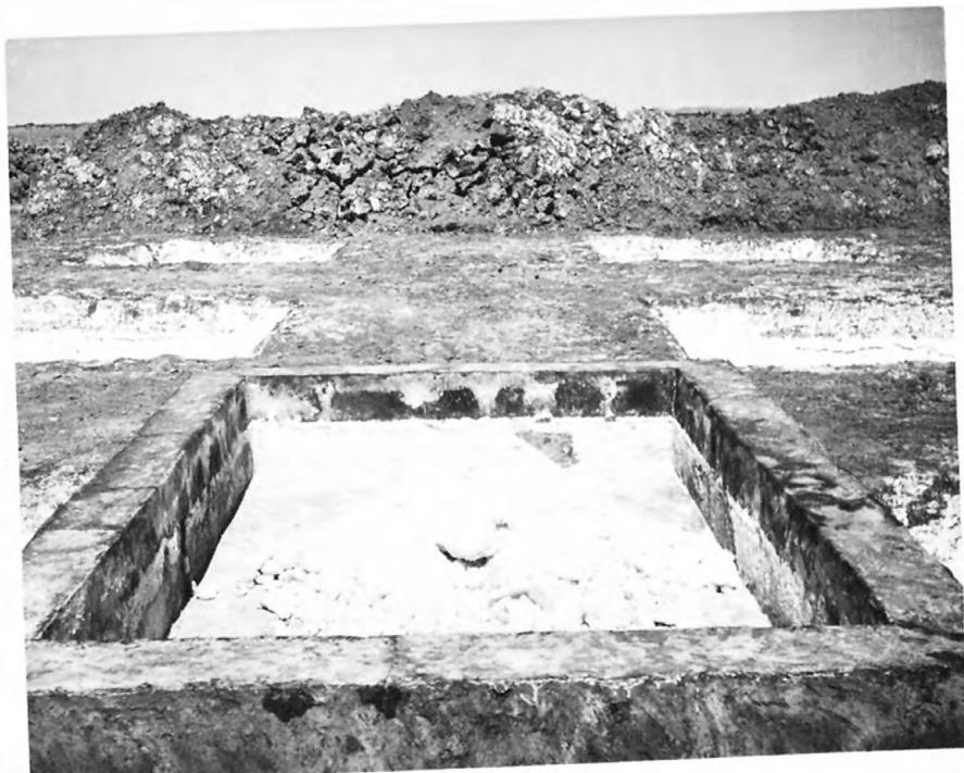
Figure 7. Evaporation to dryness was done in vats from which the crystallized salts were collected, weighed, and sampled for purposes of the study.
