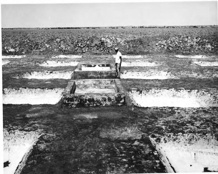
Figure 2.--Experimental plots at Edri. Crust was removed and 25 pits 3 meters square were dug to the water table.
