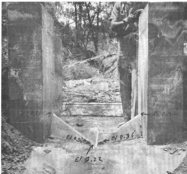
A. Upstream view showing low-water constriction
