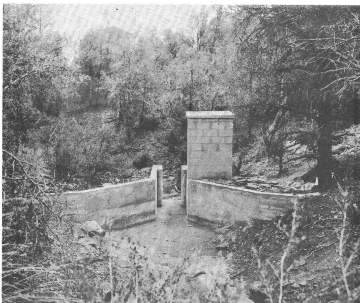
A. Downstream view of gaging station
