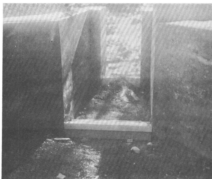
B. Downstream view of control and wooden sill
