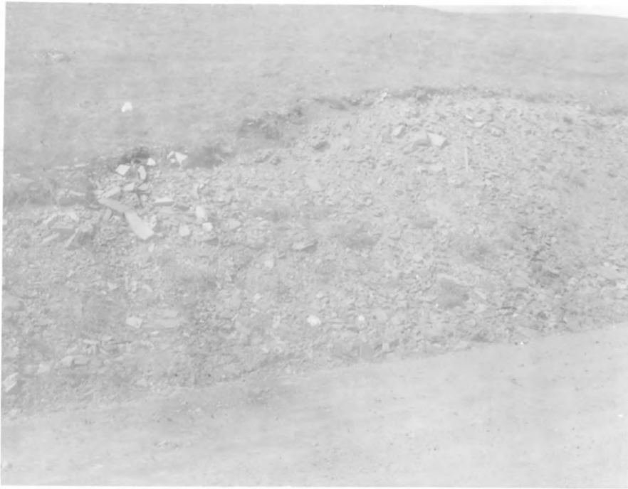
Figure 43. Road cut through a schist lithosol at Eagle Summit, Steese Highway, Alaska. The D horizon consists of schist blocks rather than bedrock; slumping of the soil over this horizon gives a false impression of soil depth in this picture. The actual depth of the solum is shown just beneath the organic mat in the center of the picture. There was no ground ice found in the solum; however the D horizon is probably frozen where undisturbed. July 5, 1960.
