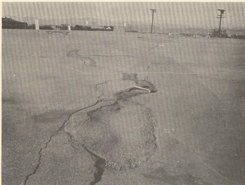
Figure 5.--Photograph showing extensive, locally broken, patching along major earth Crack I where it passes through school yard north of Overhill Drive.
