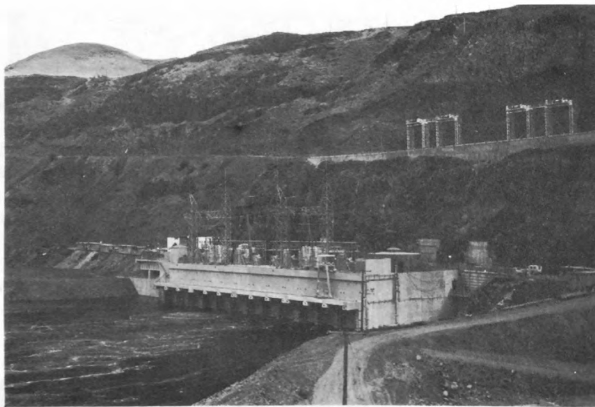
Oxbow Powerplant, Snake River, Sept. 20, 1961. Water is diverted from reservoir by a tunnel.
