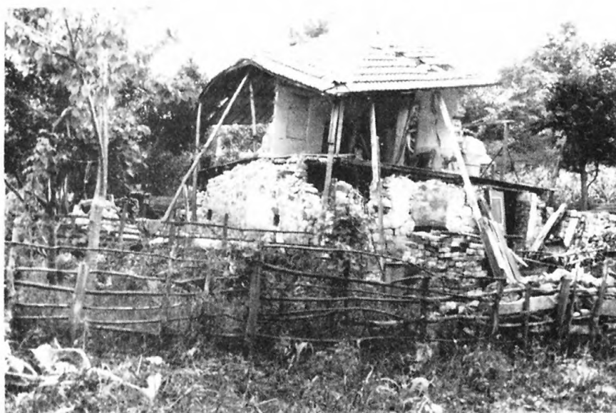
Figure 8.--Collapsed house, Çakraz Valley. Tile roof propped up after quake.
