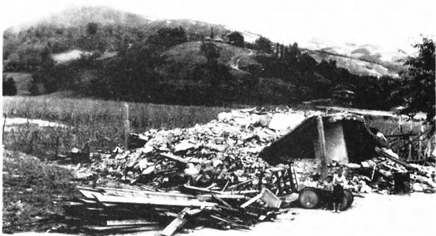
Figure 6.--Damaged house, Çakraz Valley. Approximately 100 meters to right of building in background a high minaret built on alluvium was undamaged.
