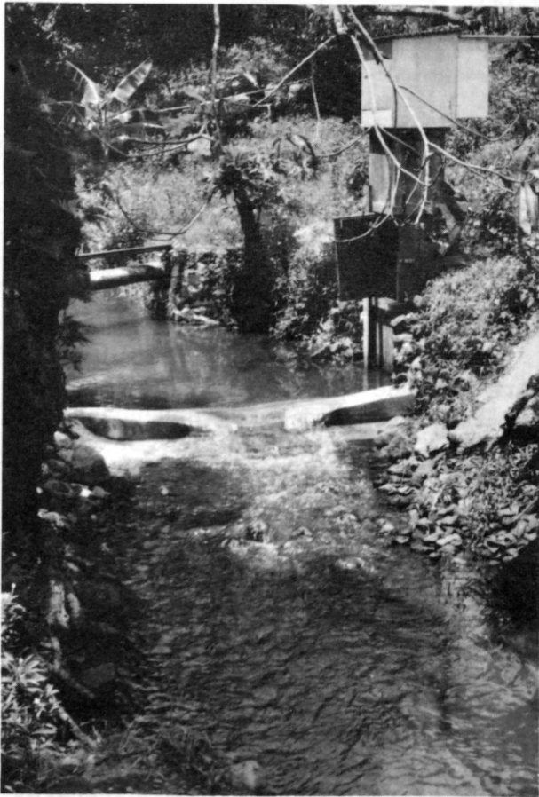
Figure 6. Artificial control, Tumunu Stream, Dublon Island, Truk Islands.
