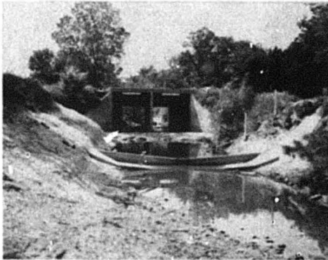
View looking upstream showing concrete control and staff gages.
