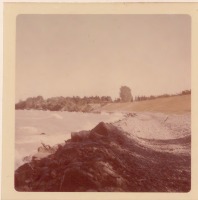
Figure 12. -- Seawall constructed to minimize shoreline erosion just east of Port Dalhousie, Ontario. EDC-010085.
