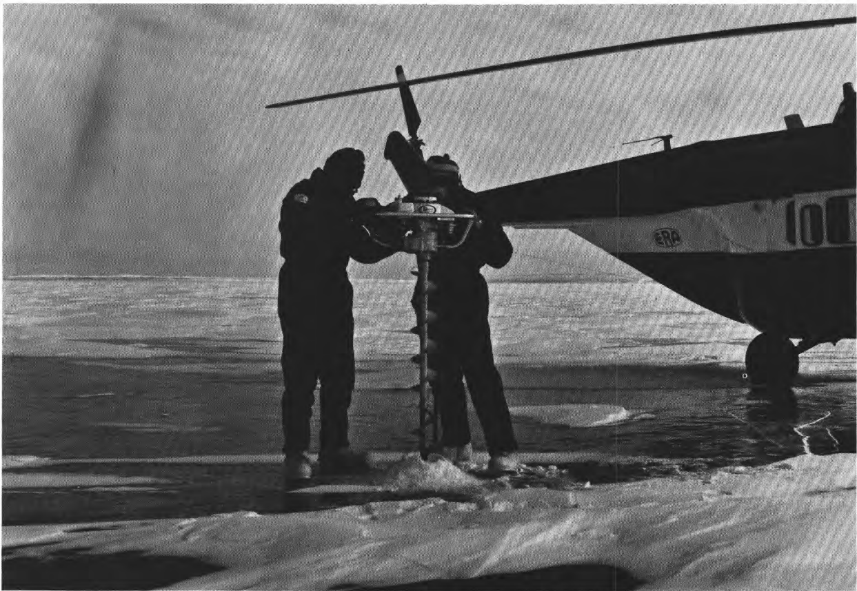
Figure 24.-- Ice drilling on the Colville River near Nuiqsut, April 25, 1975. Ice thickness is about 7.3 ft (2.2 m).
