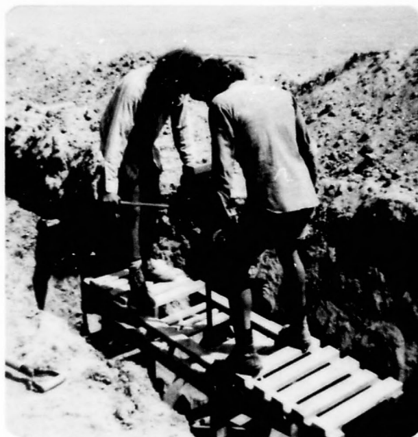
Figure 5. Drilling the pier hole.
