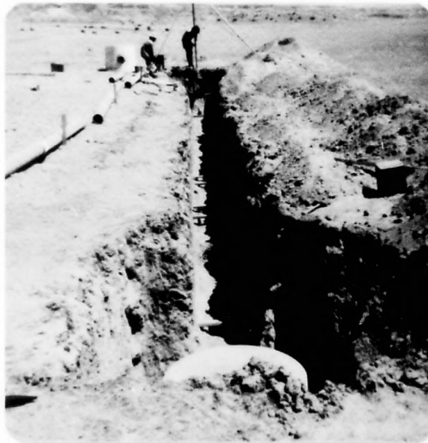
Figure 8. Beginning construction of pipe supports either side of each coupling.
