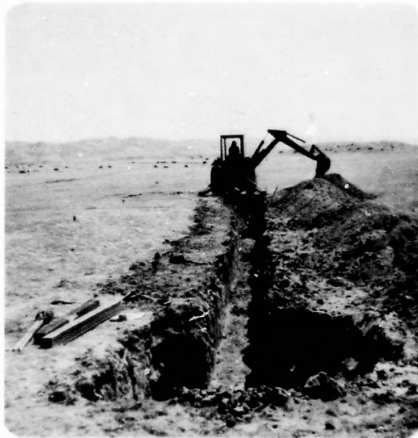
Figure 3. Backhoe operator opening up second pit at end of trench. First pit in foreground.
