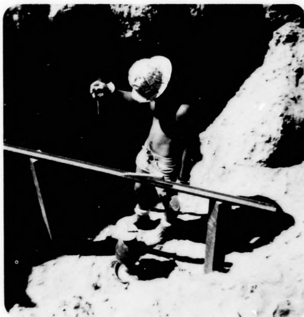
Figure 6. Instrument pier in place in grout-filled casing pipe. Rubber boot is for sealing off interior of vault from environment after enclosure is in place over pier.
