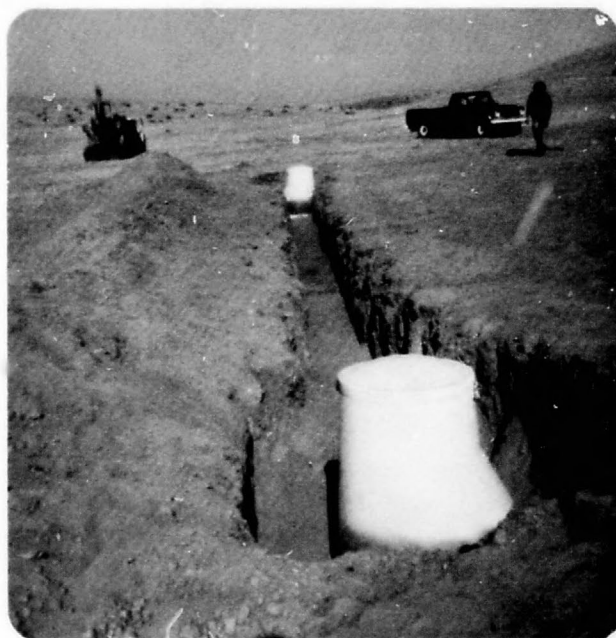
Figure 12. Top cones in place with pipe and lower enclosure already covered with dirt.
