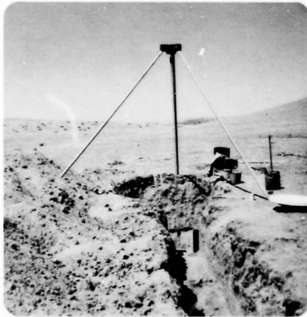
Figure 7. Block and tackle and tripod setup.
