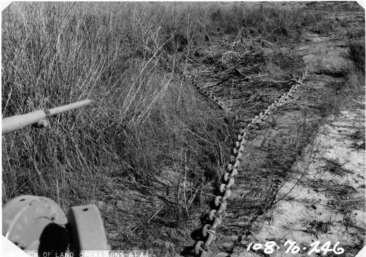
Figure 6.--Anchor chain uprooting brush killed by inundation.
