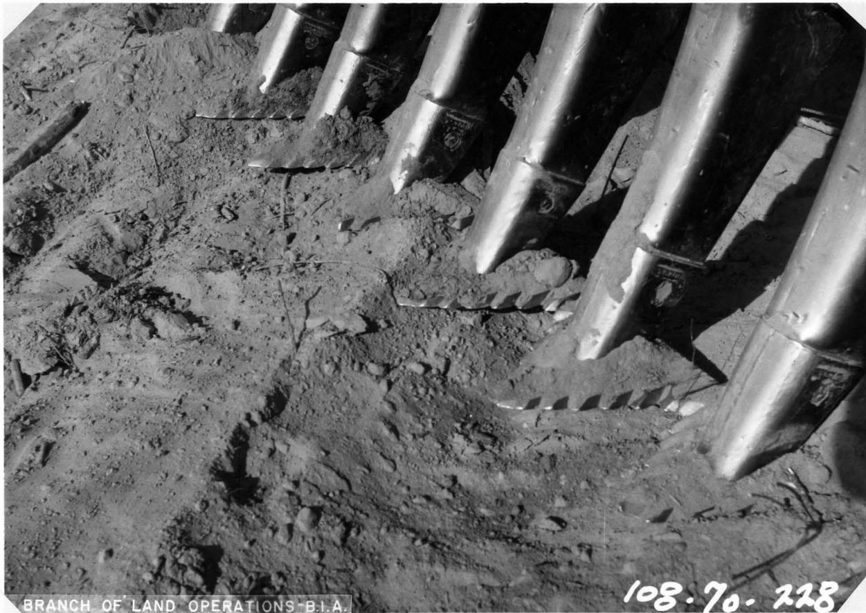
Figure 8.--Brush rake equipped with serrated points for eliminating dense saltcedar seedlings. Photograph furnished by U.S. Bureau of Indian Affairs, San Carlos, Arizona.
