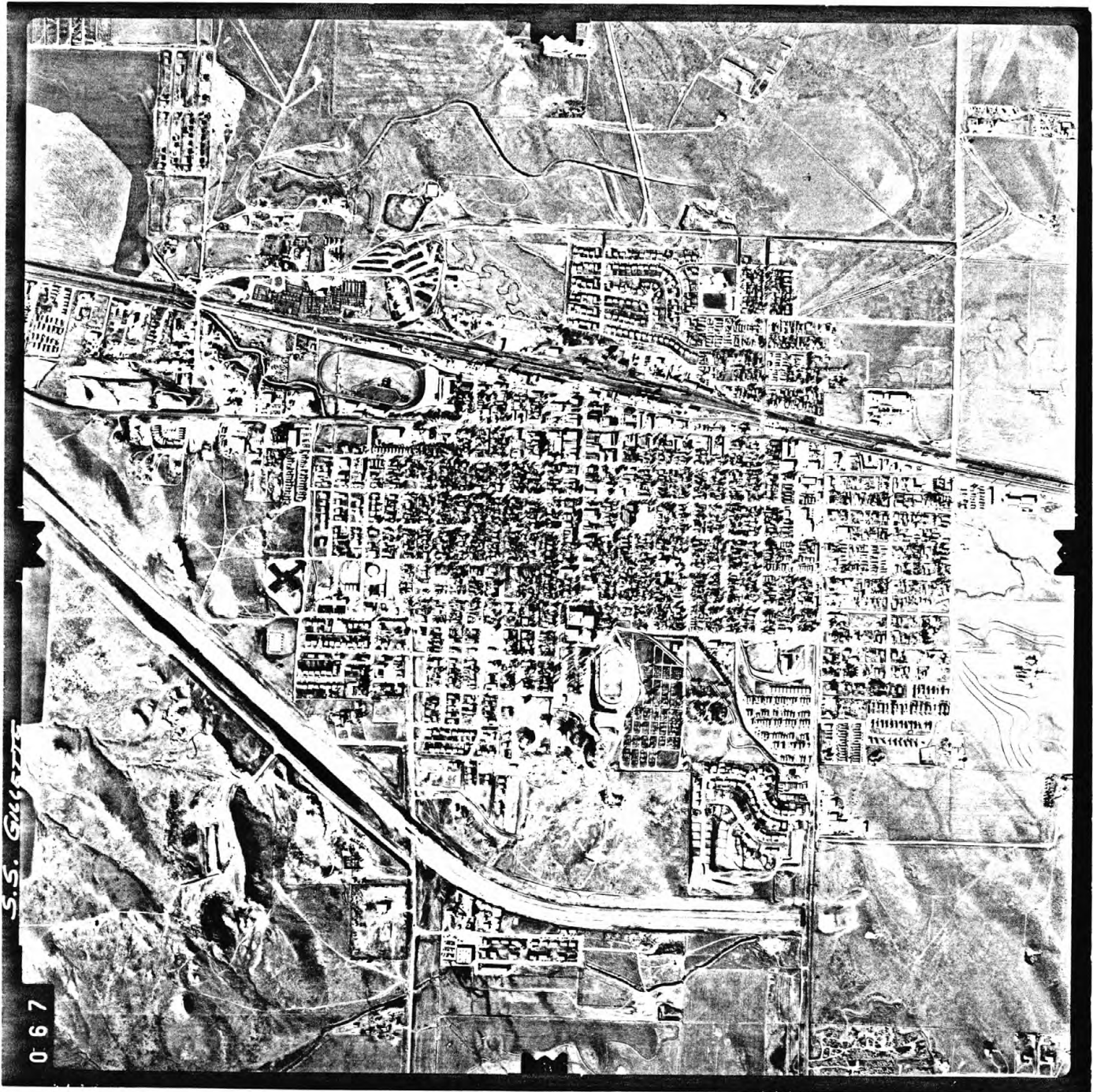
Figure 2.--Aerial photo of Gillette area in 1970
