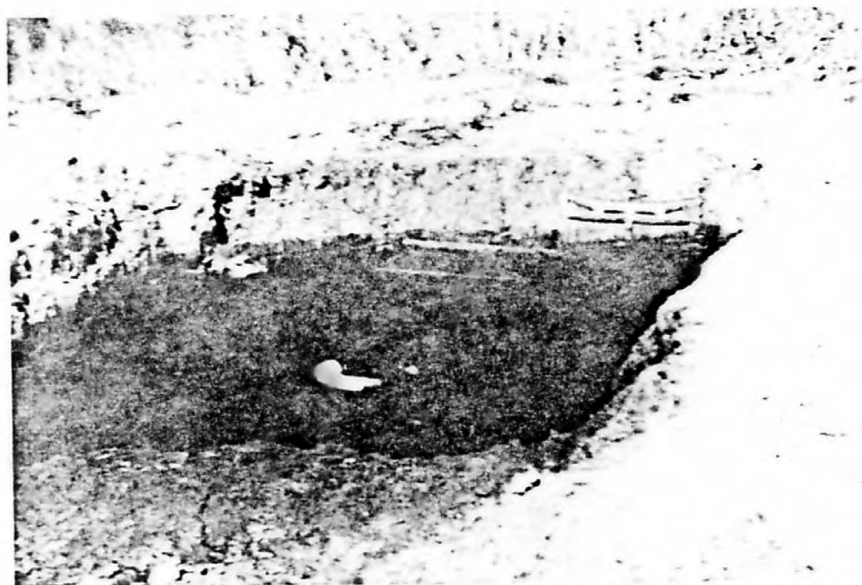
Figure 24.--Filled slurry pit at hilltop in Mayaguez landfill. This pit was filled prior to May 1975 and very little settling has occurred (January 1976).
