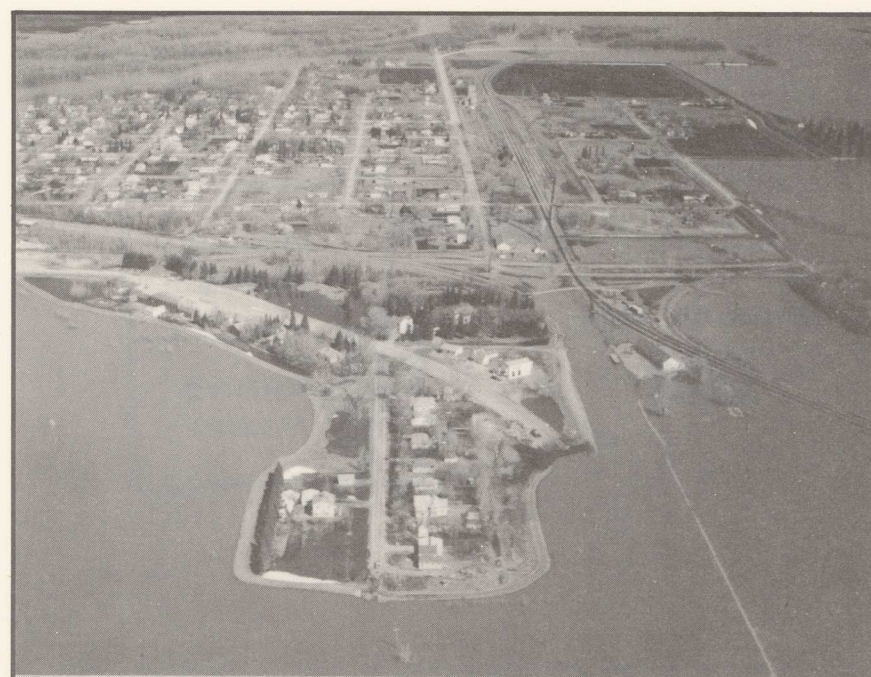
Downstream (north) view of the west side of St. Vincent, Minn.
