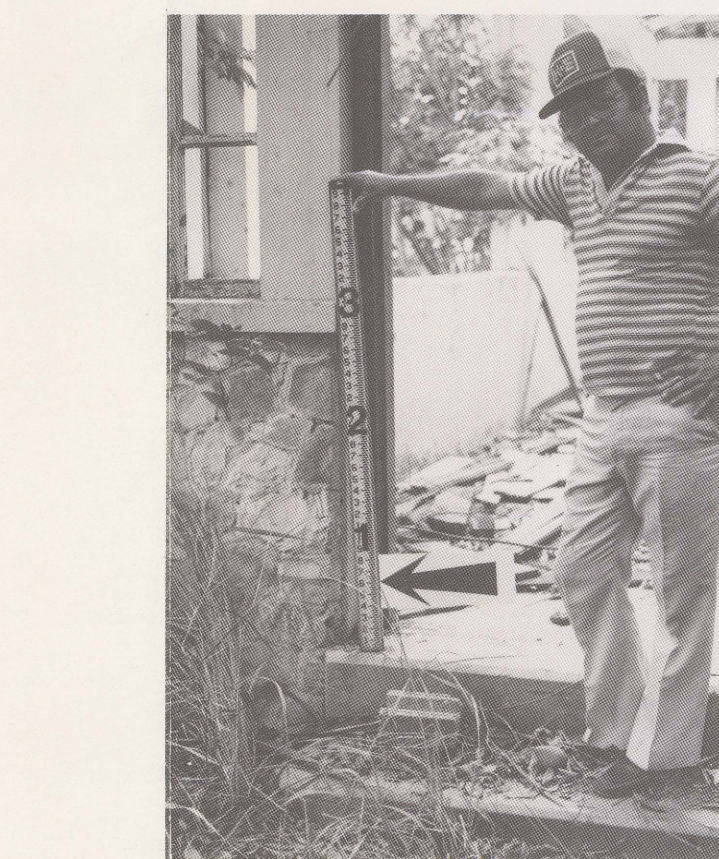
FIGURE 5. - Flood height (noted by arrow) at Central Rufina on abandoned house (photograph C).
