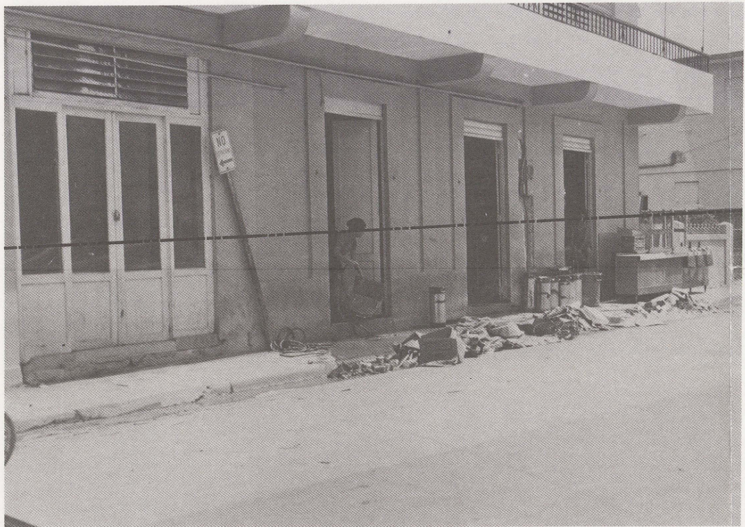
FIGURE 6.--House in front of the Utuado High School. Dashed line shows approximate flood height reached, September 16, 1975 (Photograph C).
