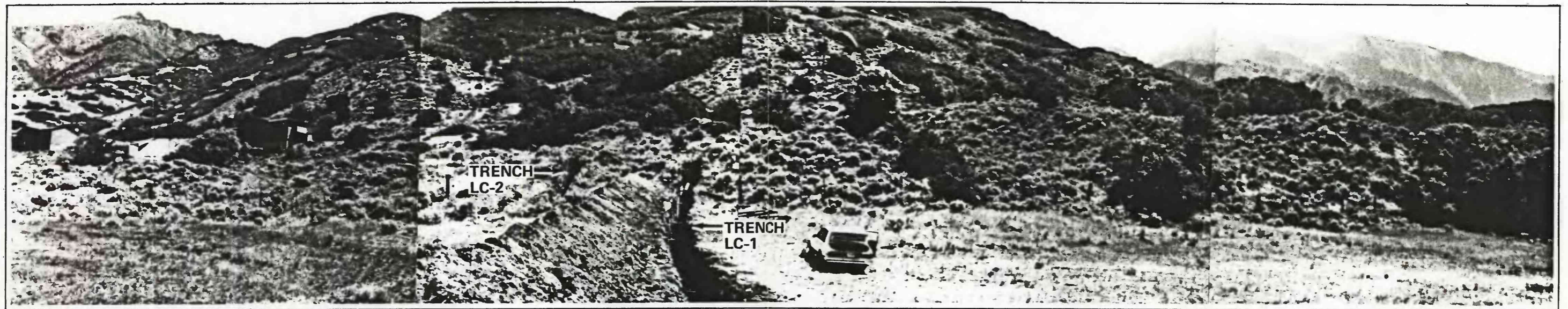
Trenches LC-1 and LC-2 were excavated across the westernmost splay of the main fault. View is east from center of graben.
