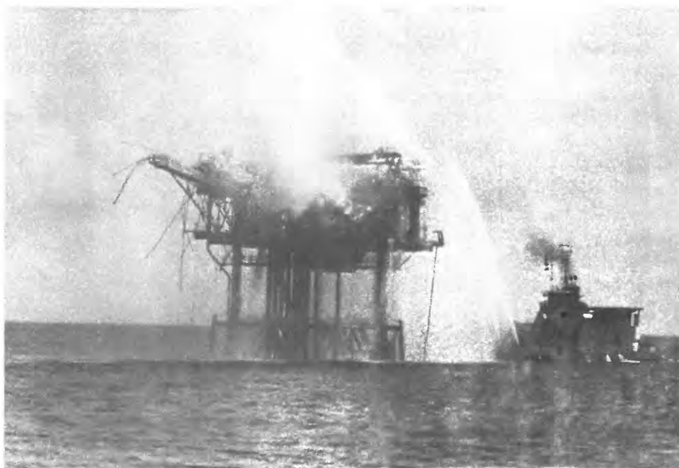
Date: After Commencement of Spraying by Jet Barge Jirafa on 8/28/80 Location: Vermilion Block 348, Platform "A" Photographer: Supplied by Mesa Petroleum Co.
