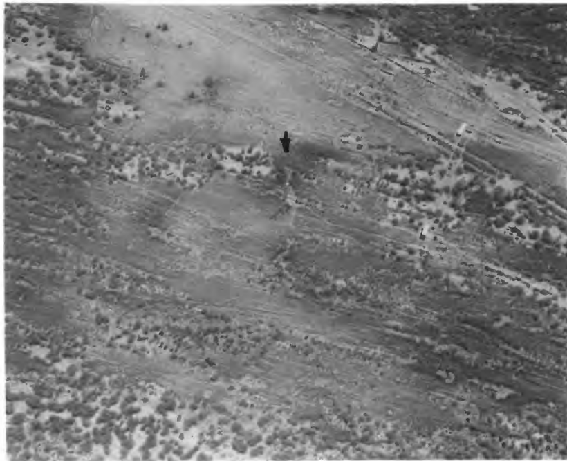
Figure 2B.--View to the south from higher altitude. Note irregular nature of planting. Instrument shack and propane tank visible to right of mast (arrow).
