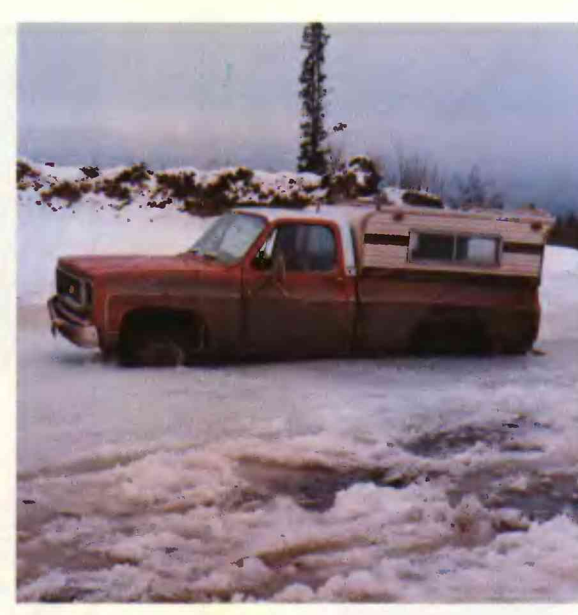
Figure 3b. -- Hazardous road conditions created by malfunctioning road drainage systems and freezing of subsequent ground-water seepage (Goldenview Drive, December 1980).
