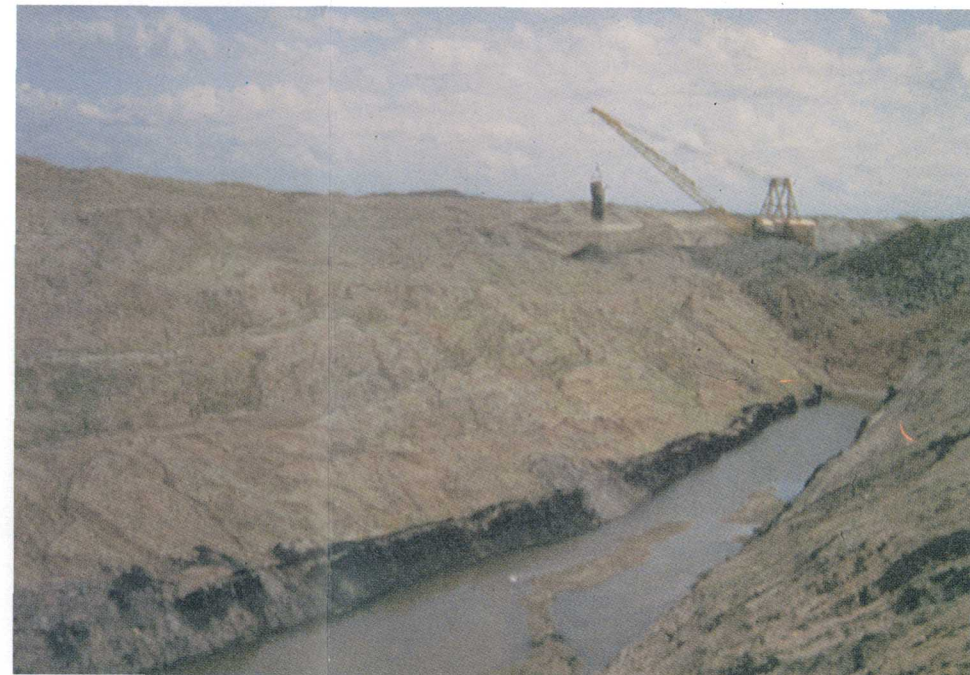
Dragline removing overburden at Velva Mine.
