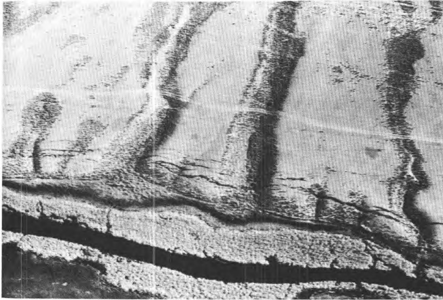
Figure 6. Oblique aerial photo of fissures along alluvial-fan fronts noted on Fig. 5. Car tracks across center of photo are about 5 ft. apart.
