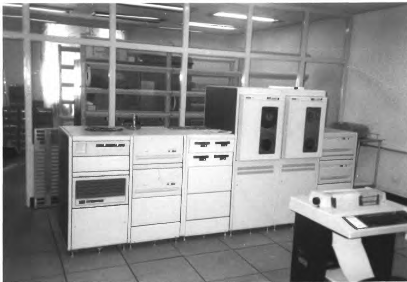
Figure 2: Data Processing System at Data Management Center
