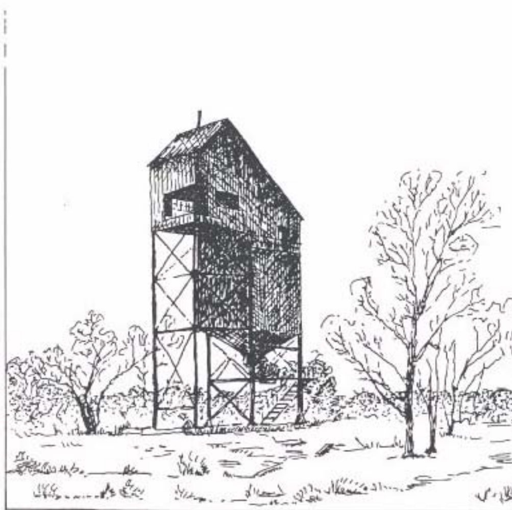
Ore loader in the Tar Creek area
