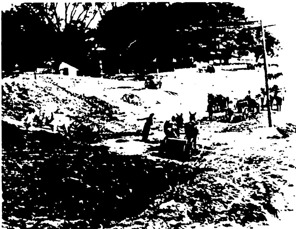
Figure 1. Levees were constructed with mule teams and drags, a system that was discontinued, but used to construct this Jefferson Parish levee, ca. 1908 (photograph courtesy of the U.S. Army Corps of Engineers, New Orleans District).
