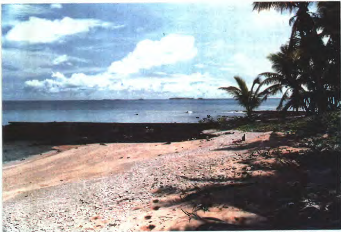
Plate 17. Rusted remnant of a WW II landing platform along a lagoon shoreline, Ulithi Atoll. Note the unconsolidated carbonate beach sand and gravel to the east (foreground) and winnowed rubble pavement to the west (background) of the platform.
