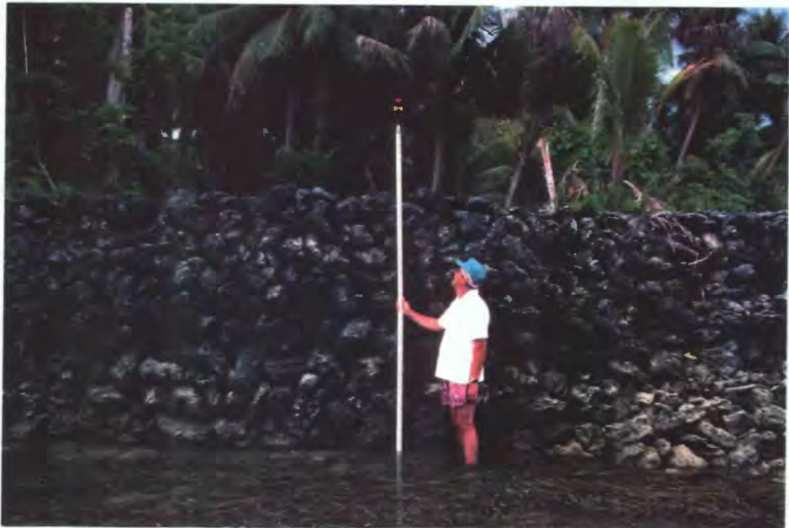
Plate 19. A traditional Yapese seawall (Gilfith, SW Yap Island) constructed mostly of hand-fitted coral blocks. Individual coral heads are collected from the reef and used in walls to both protect the shoreline and reclaim land.
