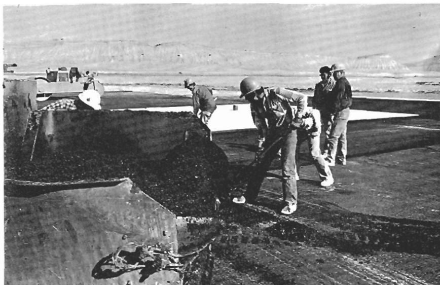
Potassium, uranium, and thorium calibration pads for radiometric measurement equipment were completed at Grand Junction's Walker Field airport.
