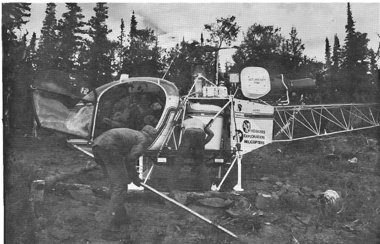
Drilling and logging of boreholes in areas of southeast Wyoming were accomplished by transporting equipment with helicopters.
