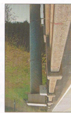
Typical flood-monitoring gage composed of a water stilling well and a gage house that shelters stage-recording equipment atop the stilling well. Gages are normally mounted to bridges where the river stage data are transmitted to the Georgia District Office in Atlanta.
